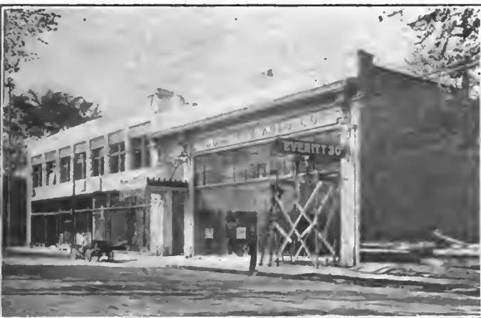
Everitt "30" Dwells In a Well-Equipped Building, as Shown
